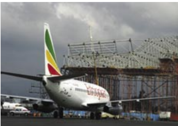
From top to bottom: Line engine maintenance, New maintenance hangar under construction, Spray services in the Sudan, working on customer aircraft and engine overhaul.
